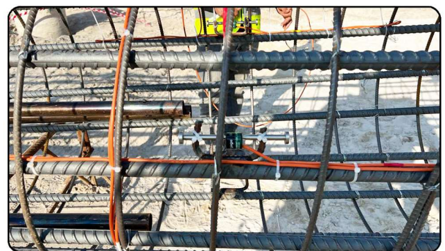
[Model 1240 installation in cage of pile load test]
