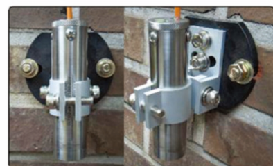
[Installation of VW inclinometer]
