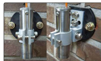
[Installation of VW inclinometer]
