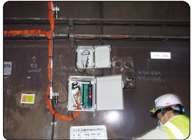
[ADL-16V Installation in tunnel]
